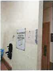
Women's Restroom Drywall prep/repair
