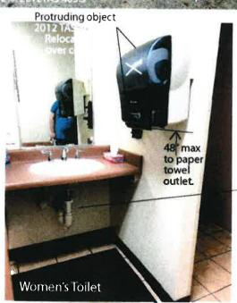
Protruding object 2012 TAS 204/307. Relocate PTD over counter
